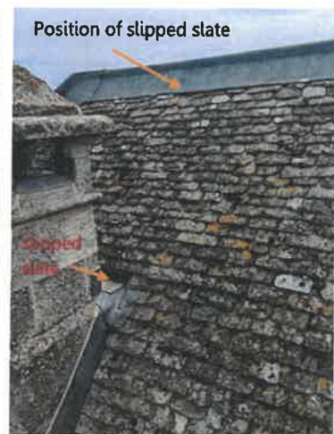
3. W roof slope
