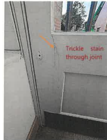
21. Fire escape door to office
