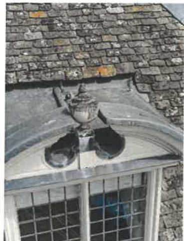
12. N Dorner- new urn completely bare
