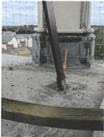
10. Clock Cupola Floor – Bell support rusting
