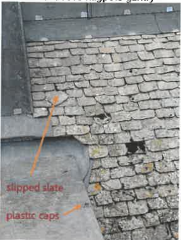
4. W roof slope
