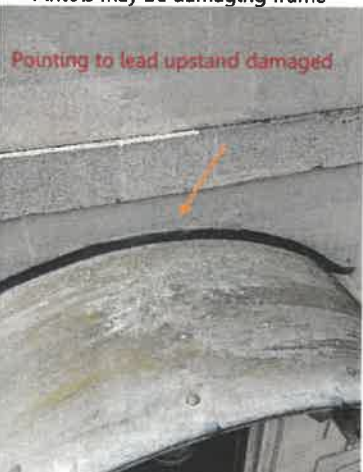
16. Lead cover to entrance canopy
