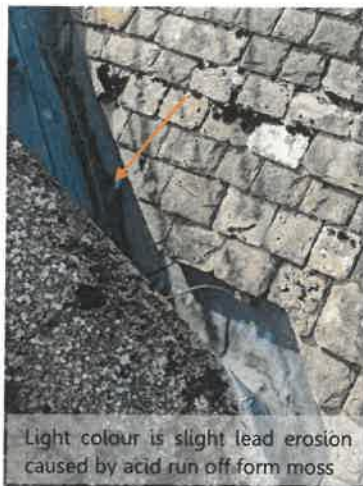
2. Lead valley to W side of N pediment
