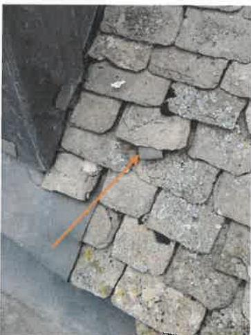
5. Slate temporarily wedged
