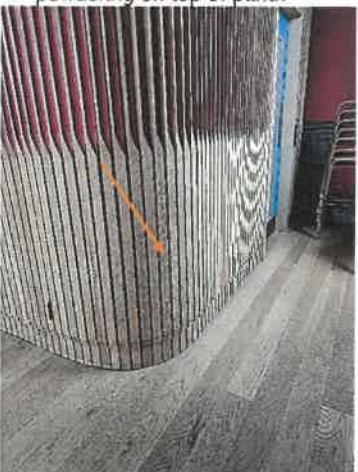
25. Slight white bloom on pod timbers on first floor
